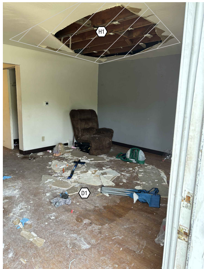
A VIEW OF GYPSUM BOARD/DEBRIS - LIVING ROOM
